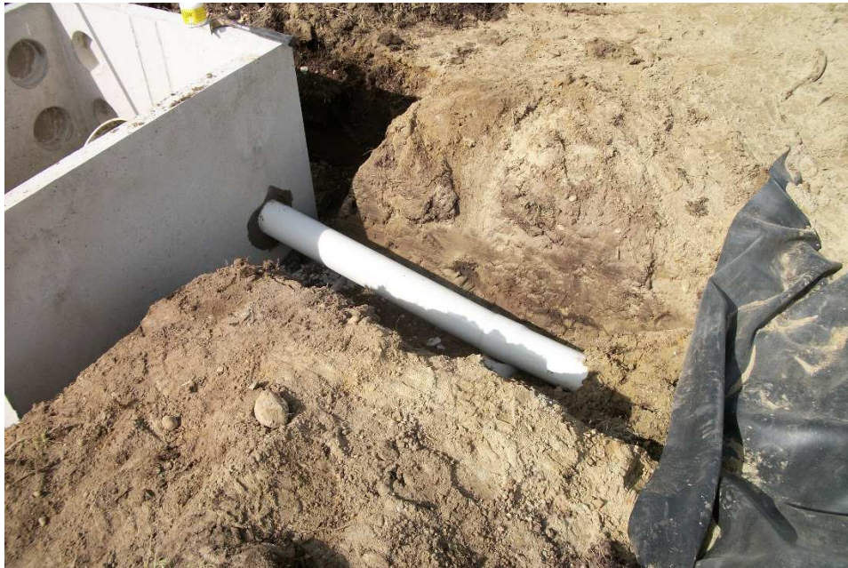
Figure 10: Connecting inlet pipe to inlet box. (John Scandrett).
