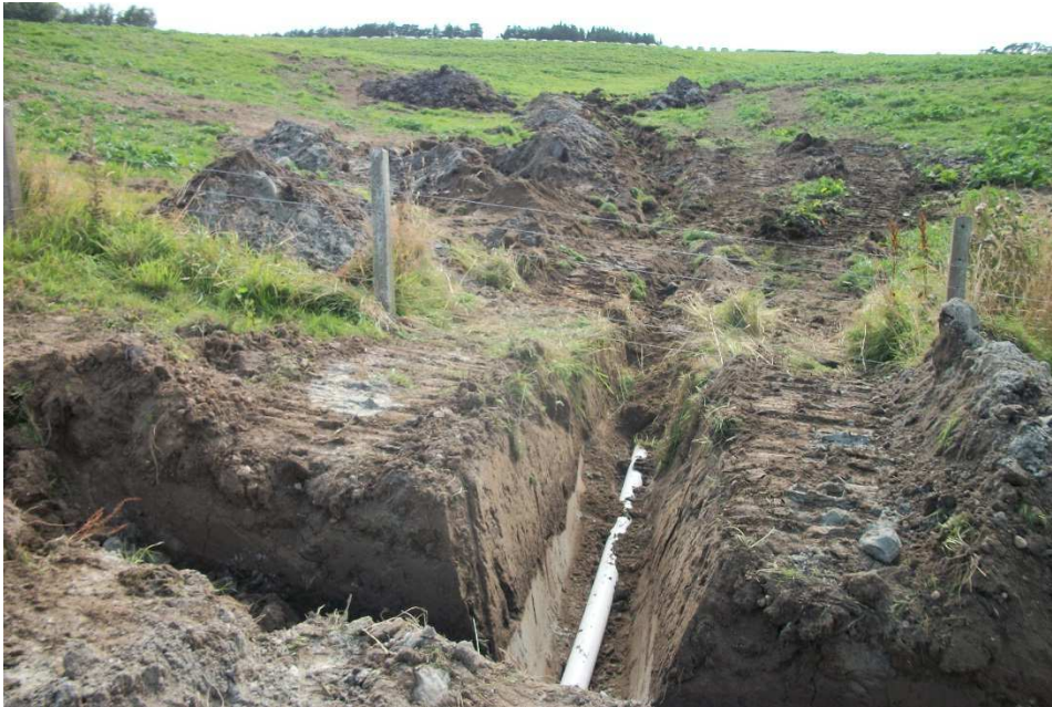
Figure 11: Inlet tile drain replacement and grading. (John Scandrett).
