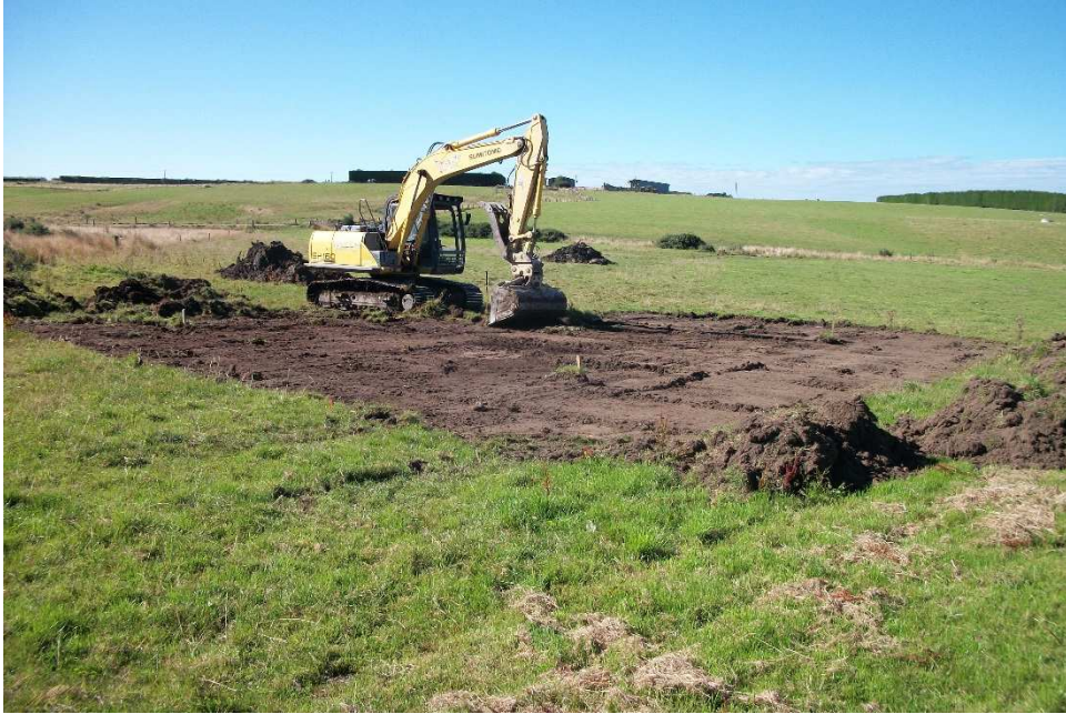
Figure 5: Topsoil removal. (John Scandrett).
