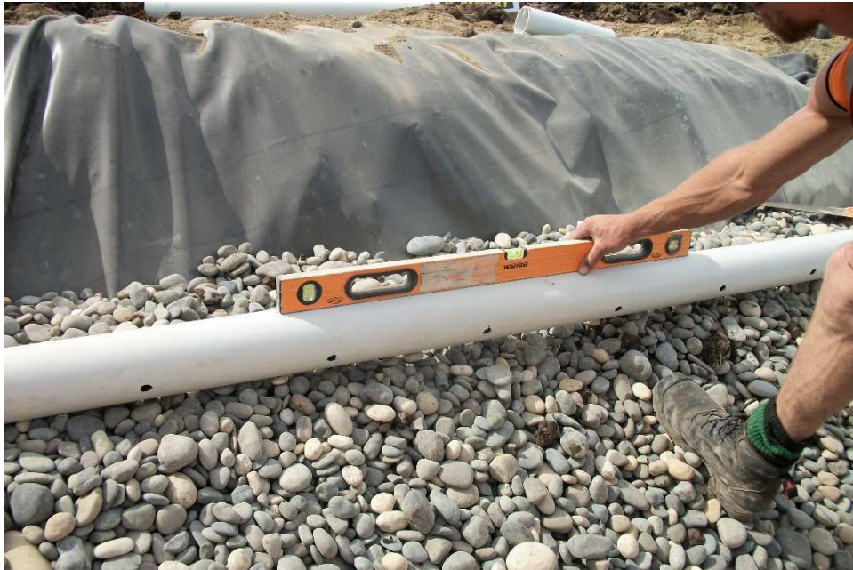
Figure 9: Levelling inlet distribution gallery. (John Scandrett).
