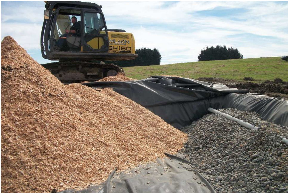
Figure 12: Adding woodchips to the pit. John Scandrett.
