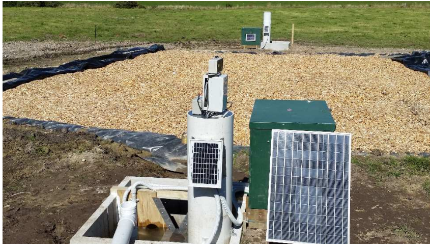
Figure 15: Inlet, outlet and complete monitoring installations. The float is inside the well (large vertical pipe with small solar panel) with encoder and NEON logger on top. Automatic samplers are stored in the green boxes. (Evan Baddock, NIWA).
