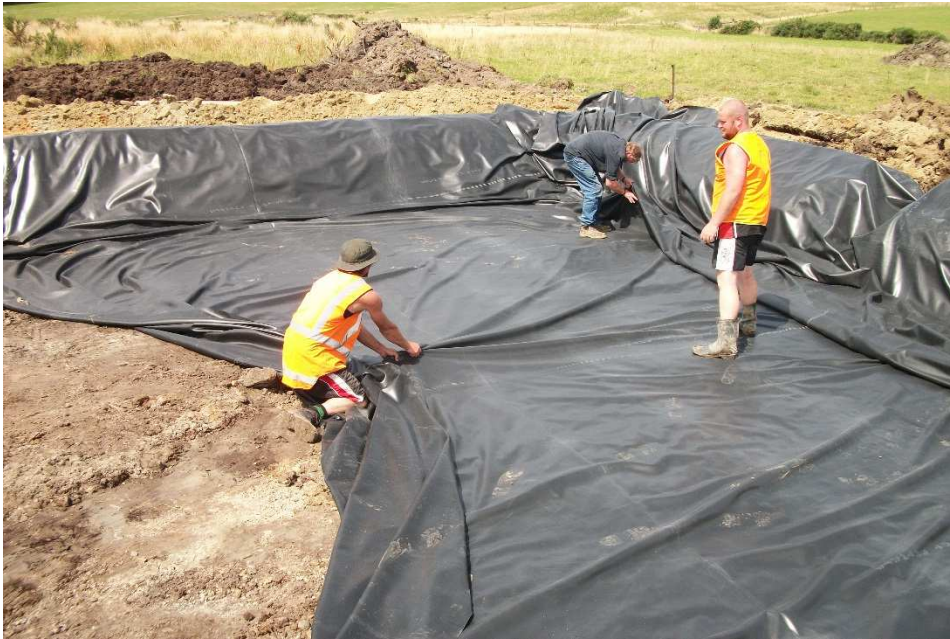
Figure 7: Liner installation. (John Scandrett).
