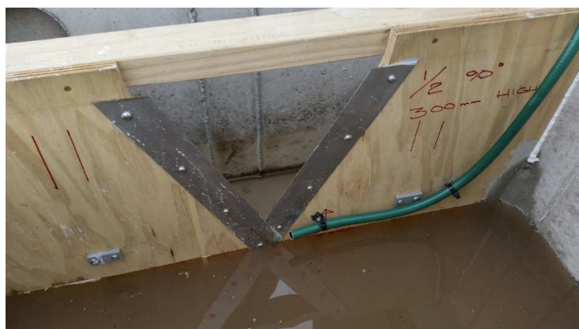
Figure 14: Inlet weir and sampler intake during construction. (Evan Baddock, NIWA).
