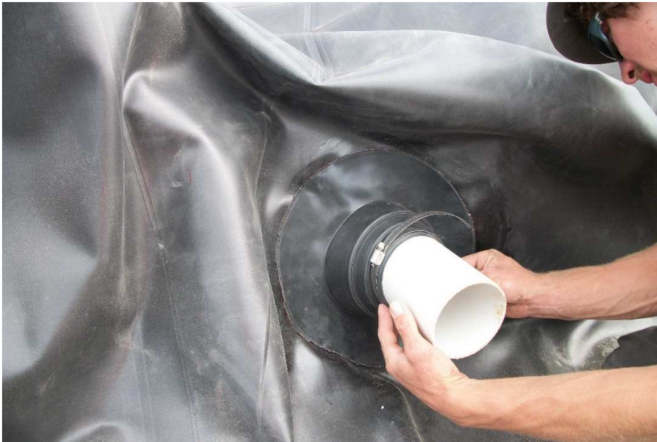
Figure 8: Securing liner boot onto inlet pipe. (John Scandrett).
