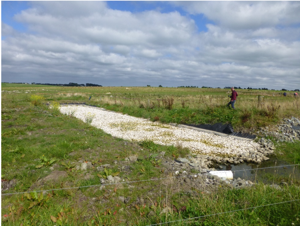
Figure 5: Oyster shell filter, with inlet in the foreground. (March 2015). (Credit: Chris Tanner, NIWA).
