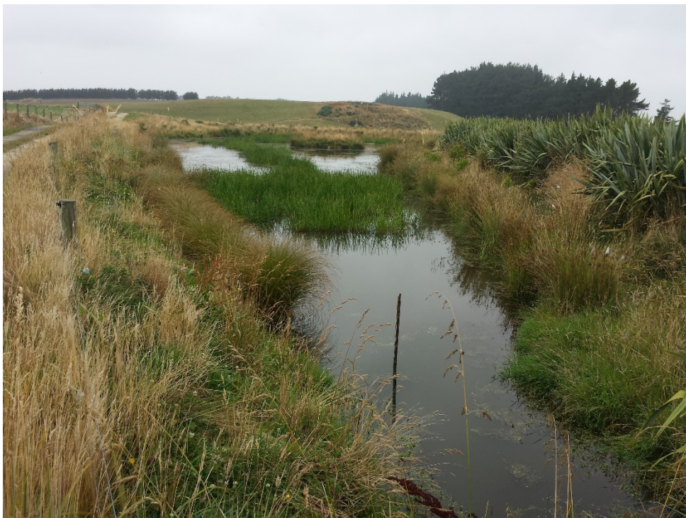
Figure 4: Constructed wetland looking from inflow end. Surface flow wetland planted with the native tall spike rush, kuta ( Eleocharis sphacelata ). (Credit: Aquatech/Environment Southland).
