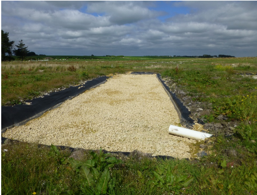
Figure 7: Limestone rock filter, with inlet in the foreground. (March 2015). (Credit: Chris Tanner, NIWA).
