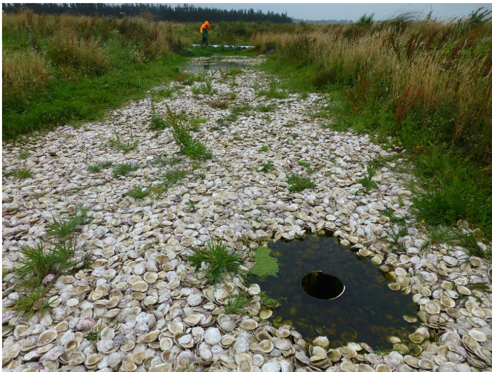
Figure 6: Oyster shell filter taken from the outlet end. The outlet is shown in the foreground. (February 2017). (Credit: Chris Tanner, NIWA). Note that the oyster shells are un-crushed.
