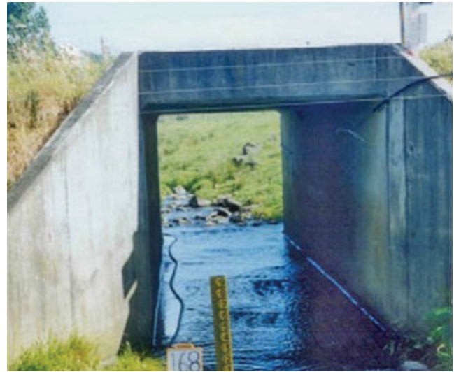
Single box culvert.
