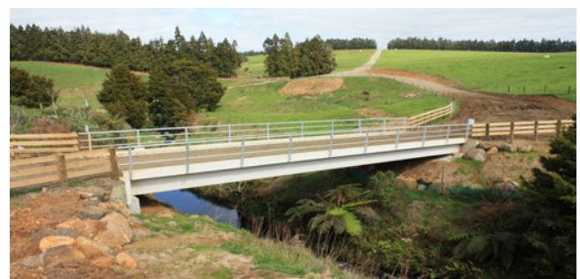
Good practice single span farm bridge. (Note that the footing of the bridge is well away from the water edge at normal flow so that the natural river bank is retained under the bridge.)
