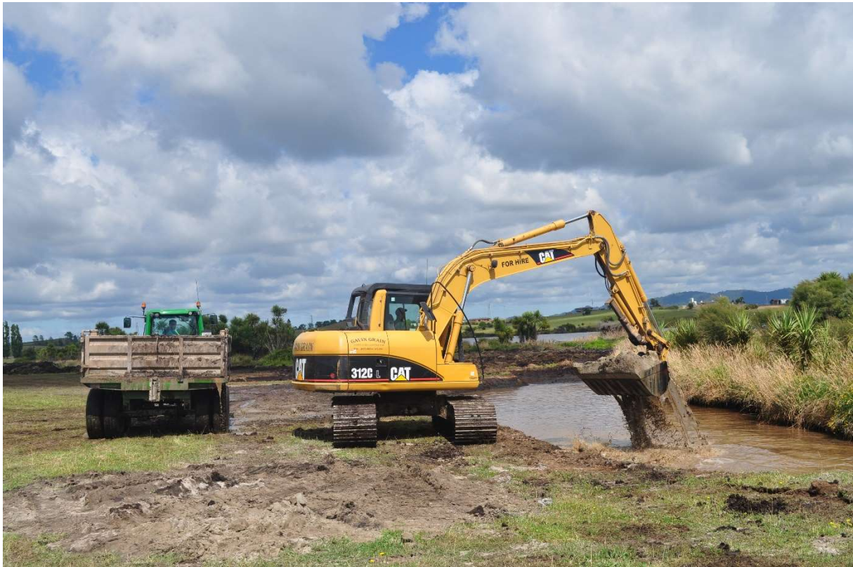
Figure 22: Emptying a sedimentation pond.
