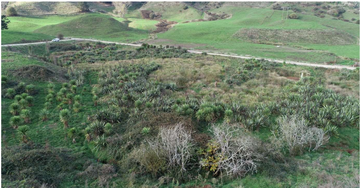
Figure 13: Example of a multi-cell wetland prior to planting. By creating multiple cells with a serpentine design, the bund height between cells is kept to a minimum. The design allows treatment of three major drain/stream inputs as well as runoff from the raceways. Use of curved edges to the wetland cells creates a natural appearance. Note also Figure 14.
