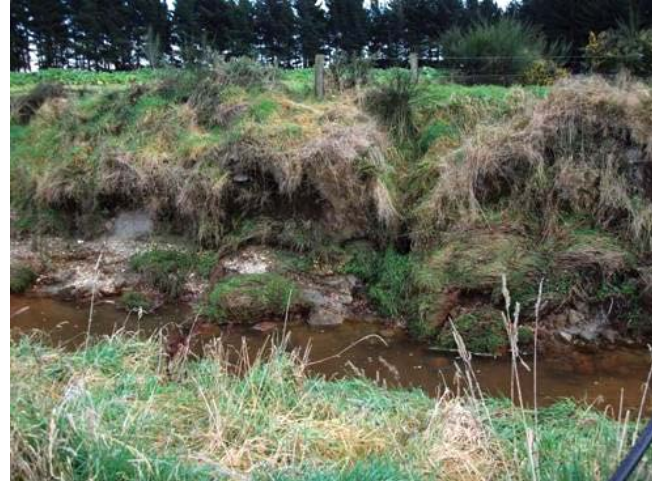
An example of moderate erosion.
