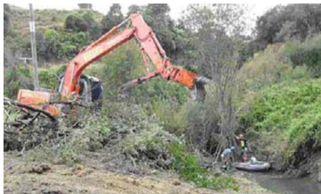
An excavator removing pest willow trees from a stream.
