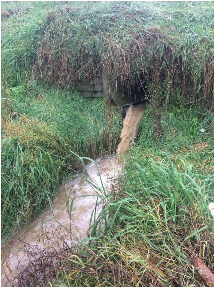
Figure 9: Input B (culvert outflow) during a storm event.
