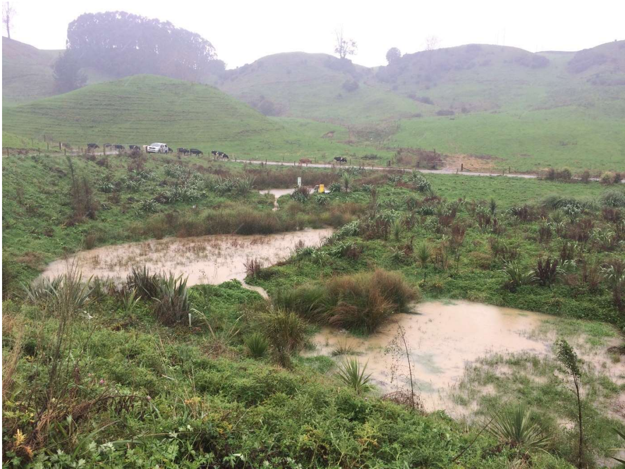
Figure 38: First three wetland cells. The first three cells operating as sedimentation basins during a high rain event.
