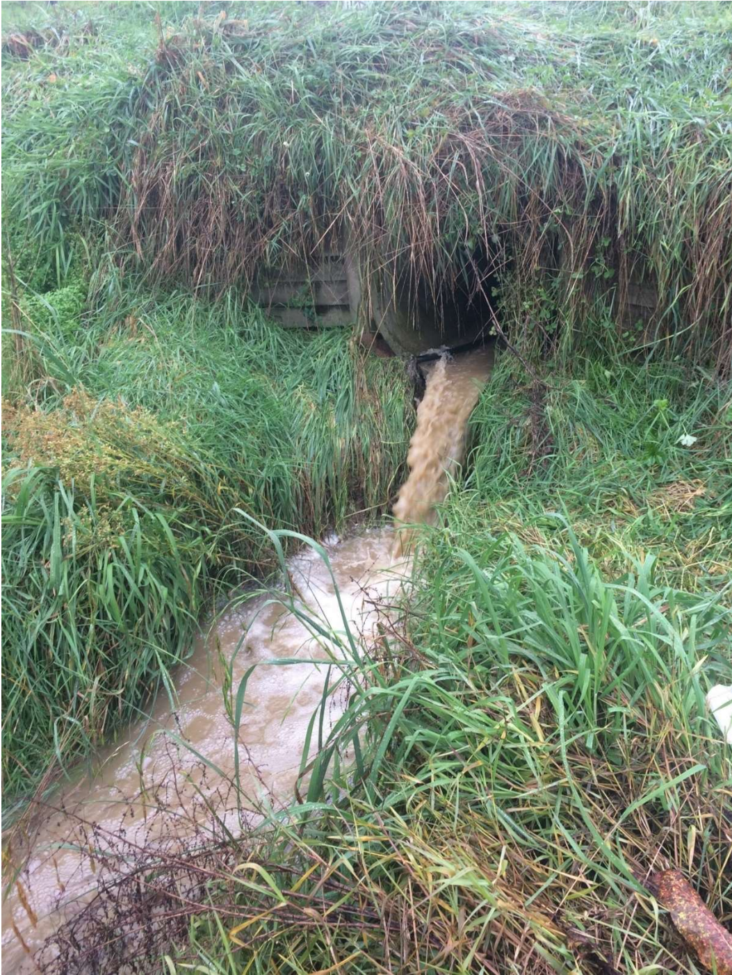
Figure 36: Inflow from culvert. The raceway runoff (Input B) carried high loads of suspended solids during rain events.
