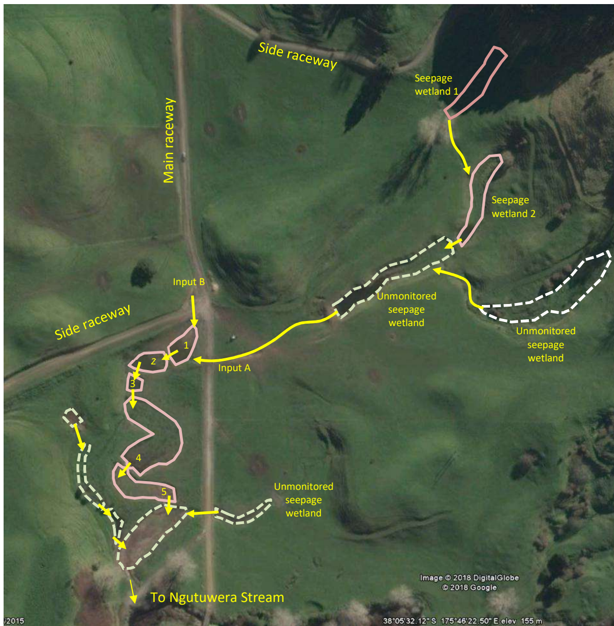
Figure 1: Individual cells of the wetland complex. Monitored locations are Input A and B, as well as the outlet from each of the constructed wetland cells (labelled 1-5). In addition, two labelled seepage wetlands were monitored. Unmonitored cells are outlined with a dashed line. Flow paths are shown with yellow arrows.
