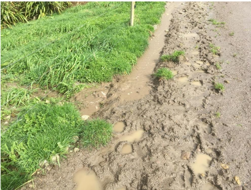
Figure 14: Contaminated flow running off east-west farm laneway and directly into cells 1 and 2. Photograph taken 13/8/19, the day after the main rain event.
