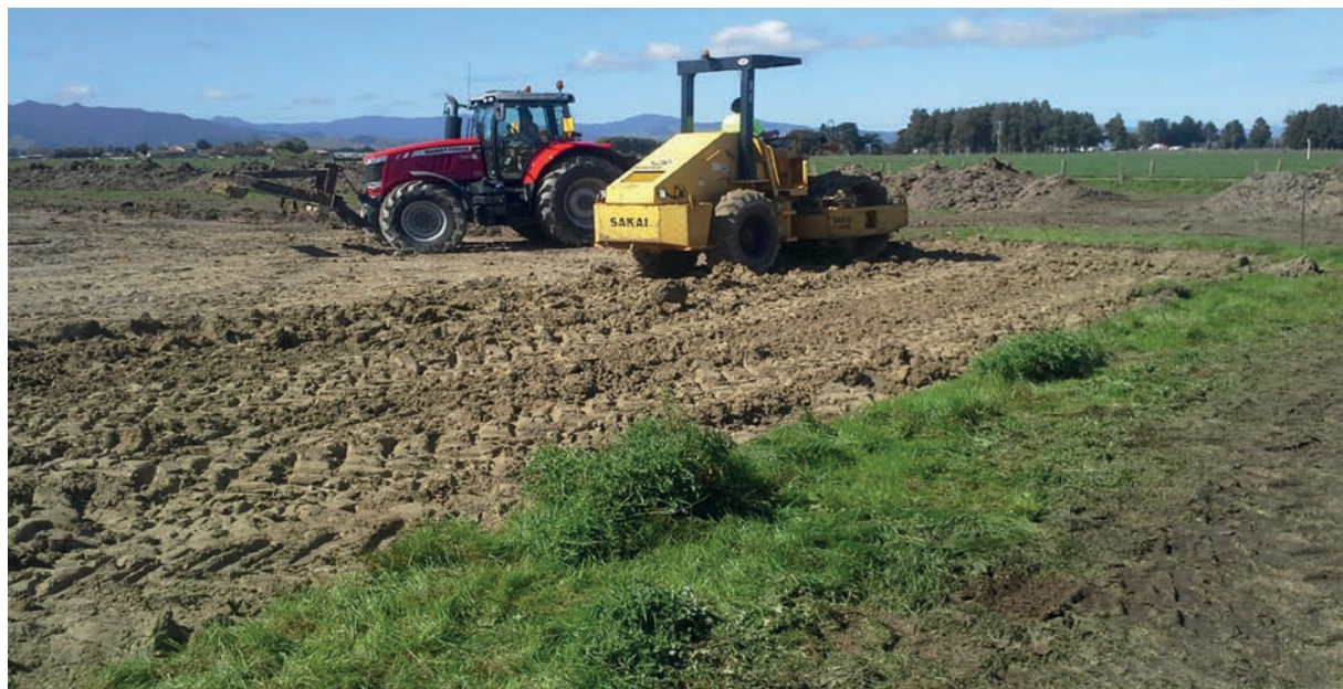
Trial Compaction Area Preparation
