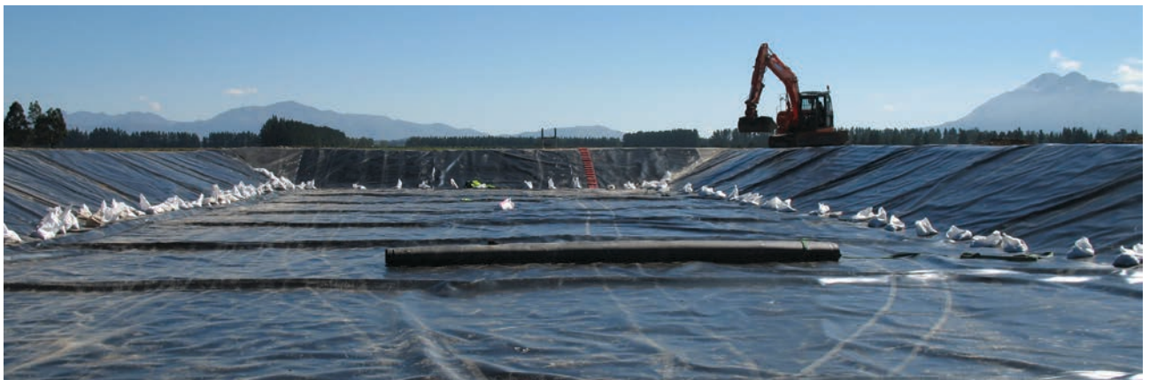
HDPE synthetic liner being installed
