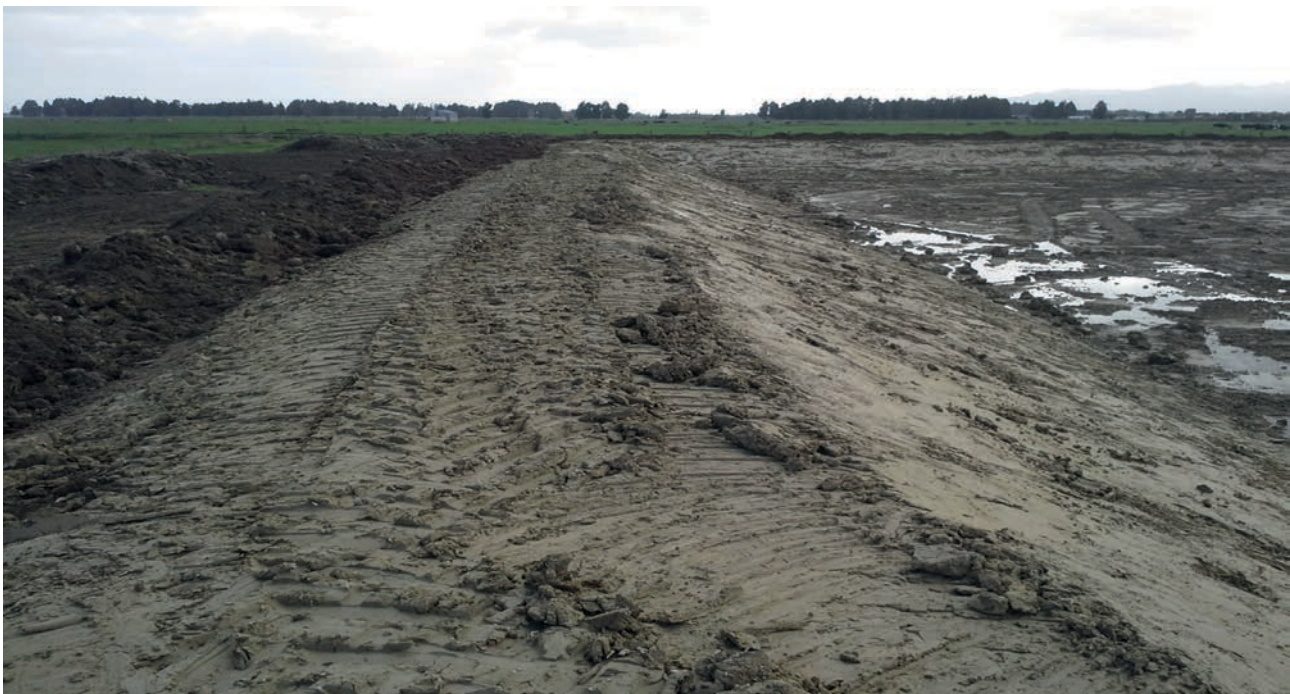
Pond Under Construction
