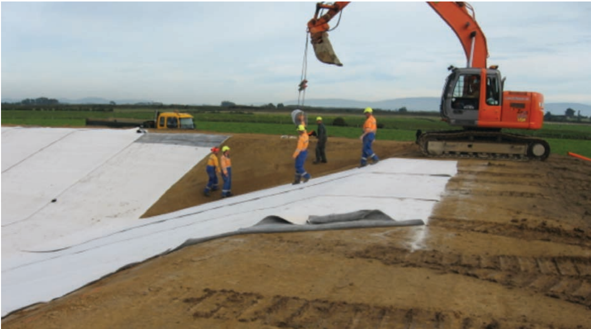
GCL liner to FDE pond.
