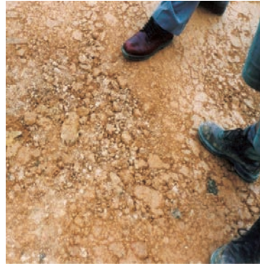
Compaction on Clay Liner
