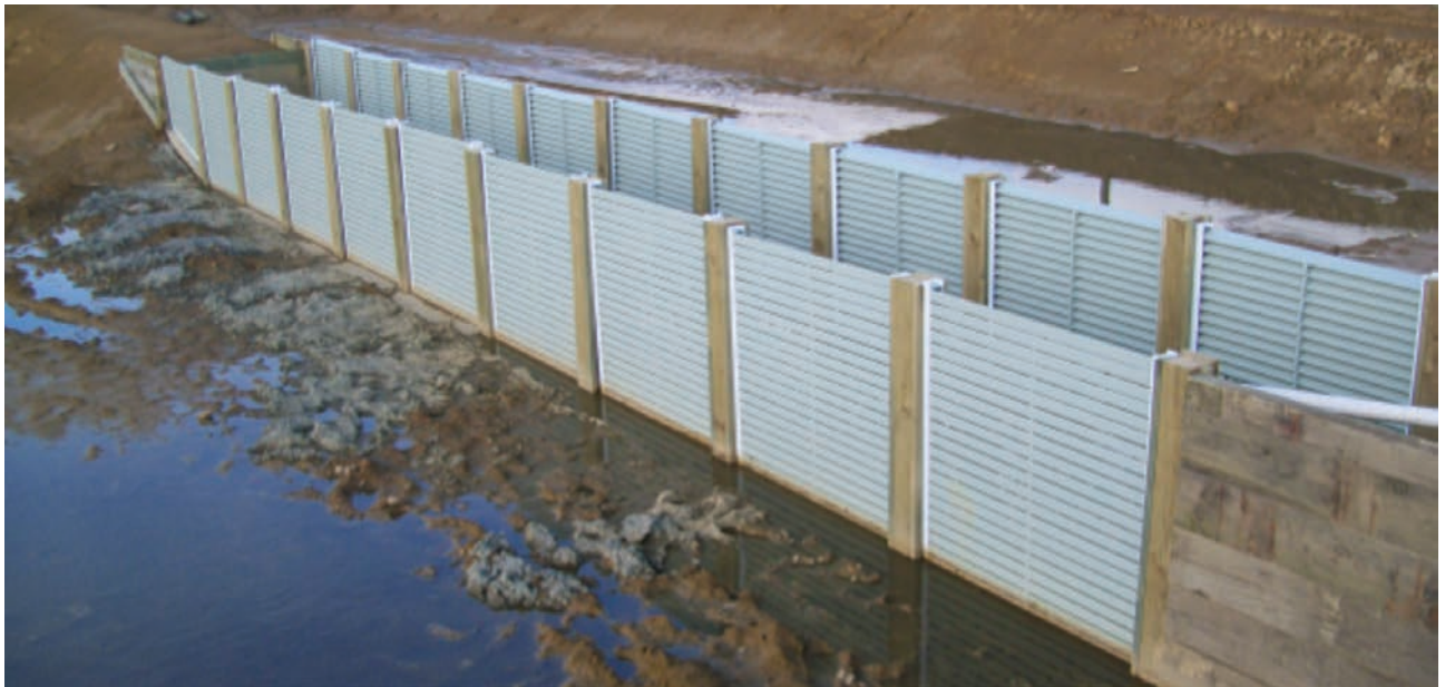
Sludge bed with double weeping wall and PVC battens
