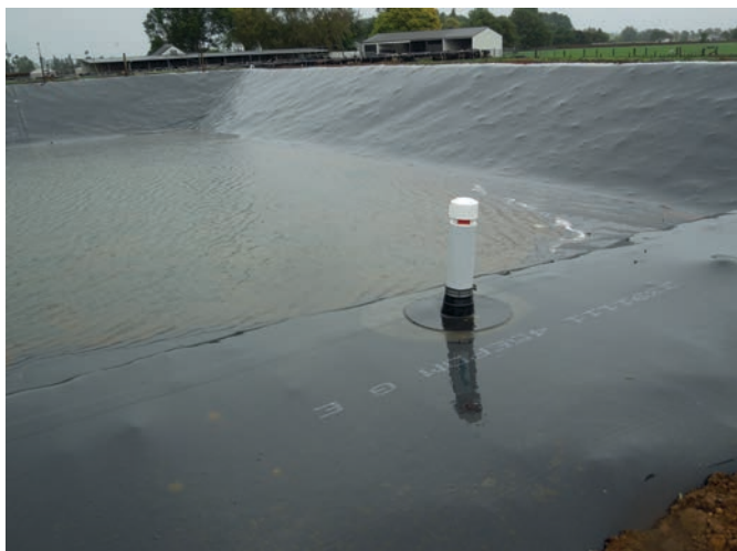
Lining with gas vent.
