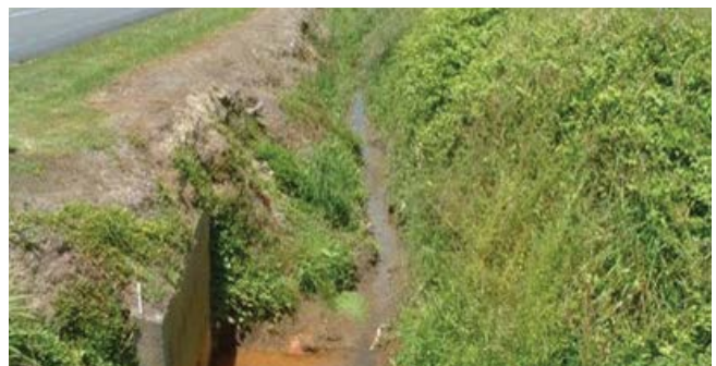
Bank erosion resulting from spraying the drain edge.
