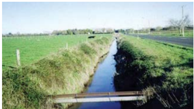
A stable drain bank fenced from stock with a grassy margin.
