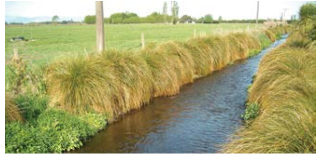
Planting shades water and helps prevent weed growth. Cleaning is made easy for a long reach digger by only planting sedges (Carex species).
