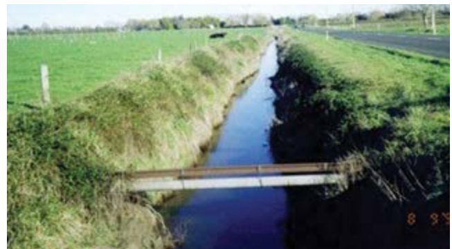
A stable drain bank fenced with a grassy margin.
