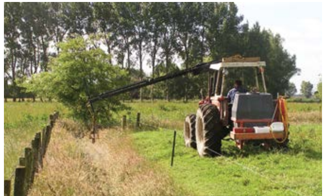
If you need to clear weeds, spray only the centre of the drain.
