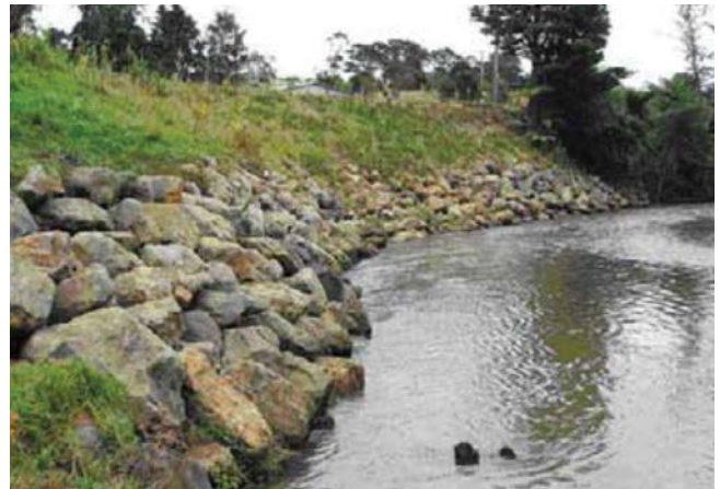
An example of an erosion control structure (rock rip rap).
