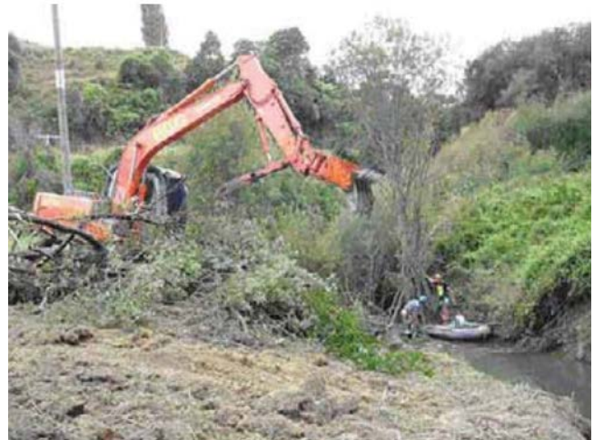
An excavator removing pest willow trees from a stream.
