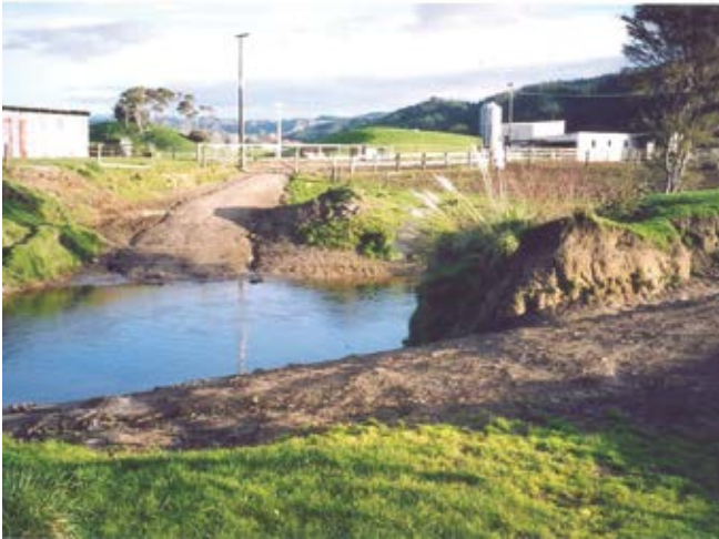
Ford crossings are entry points for sediment, nutrients and faecal bacteria. Good practice means upgrading this type of crossing to a bridge or culvert.
